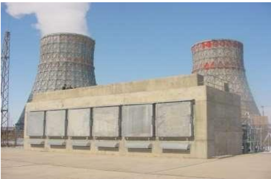
Pic. 1. External view of ANPP SNF dry storage facility
