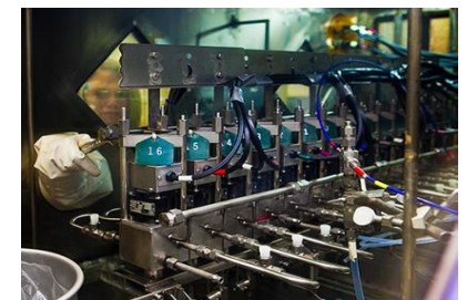
Courtesy of PNNL - Bank of 2 cm centrifugal contactors in glove box
