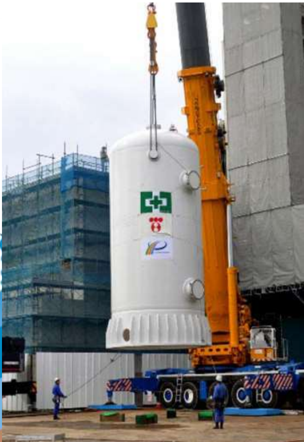
FCVS: Filtered Containment Venting System
