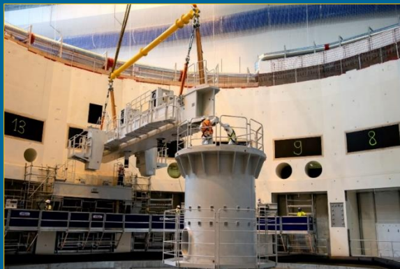
8 September 2021 – Test positioning of radial beam
