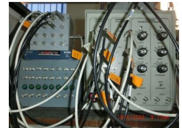
Data acquisition 5 (20 – 100 Channels)
