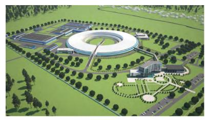
The Siberian circular source of photons (SKIF) is creating as a synchrotron radiation source with improved parameters (energy - 3 GeV, storage perimeter - 476 meters, emittance - 75 pm.mrad, current - 400 mA) in Siberia, near Novosibirsk city.
