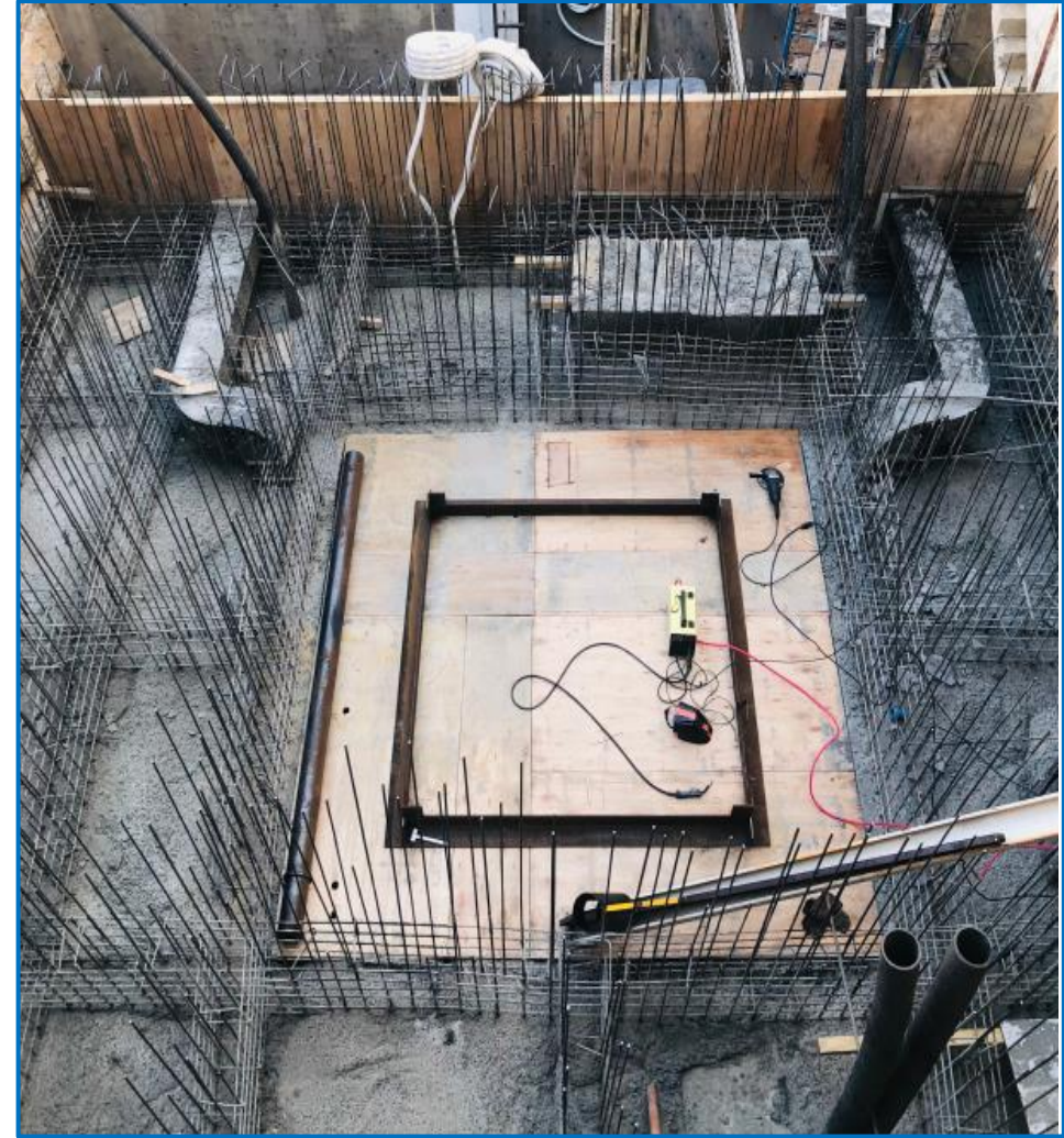
Ins and outs ventilation ducts from the vault
