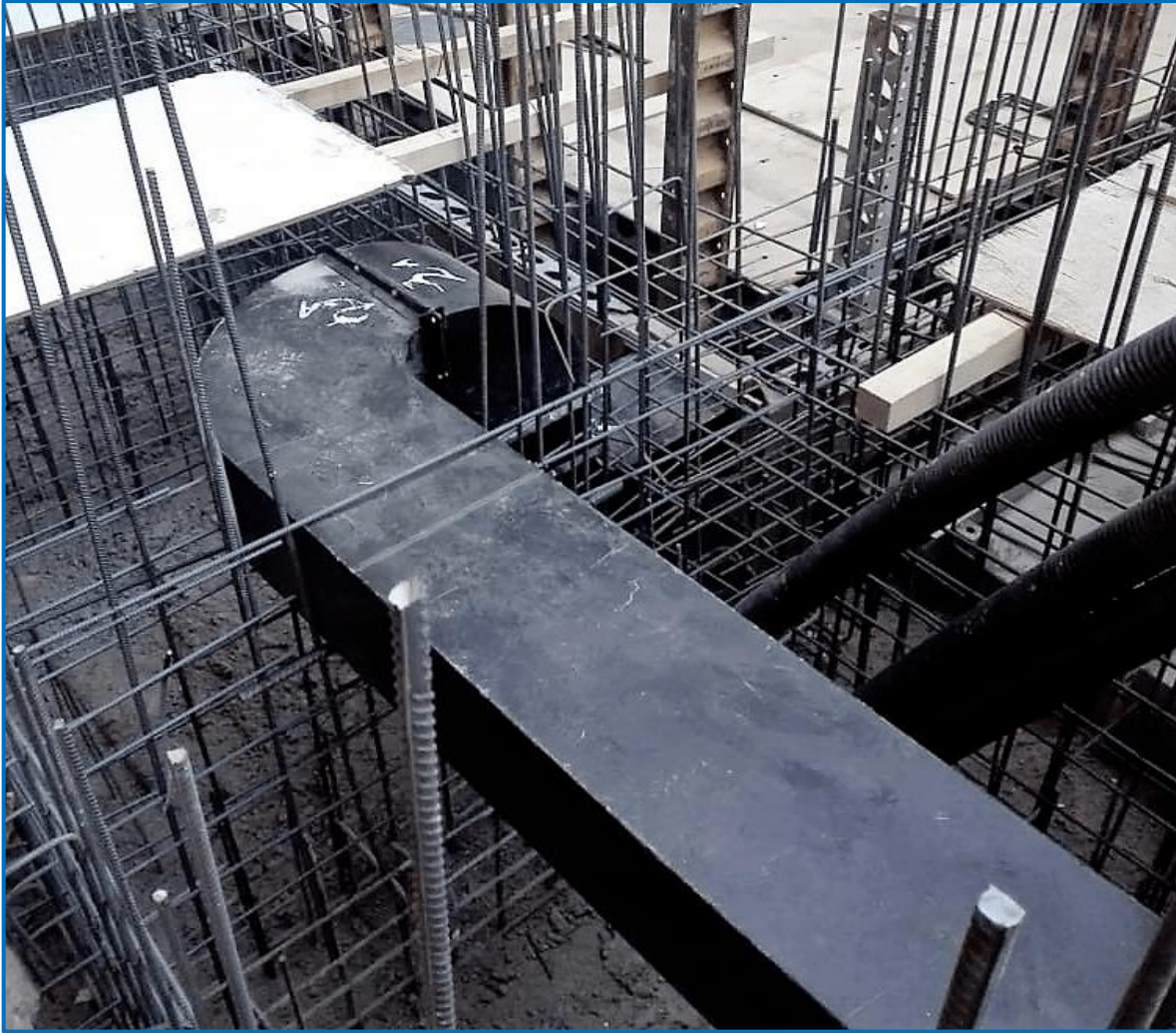
Ins and outs ventilation ducts from the vault
