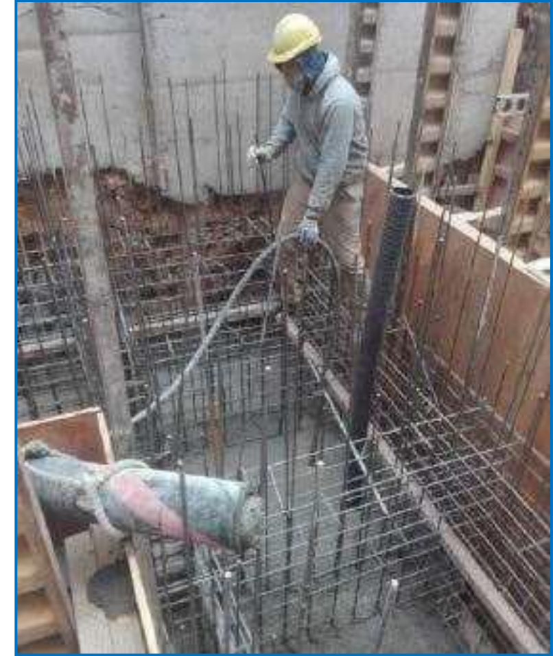
A civil worker vibrating the concrete during the cast
