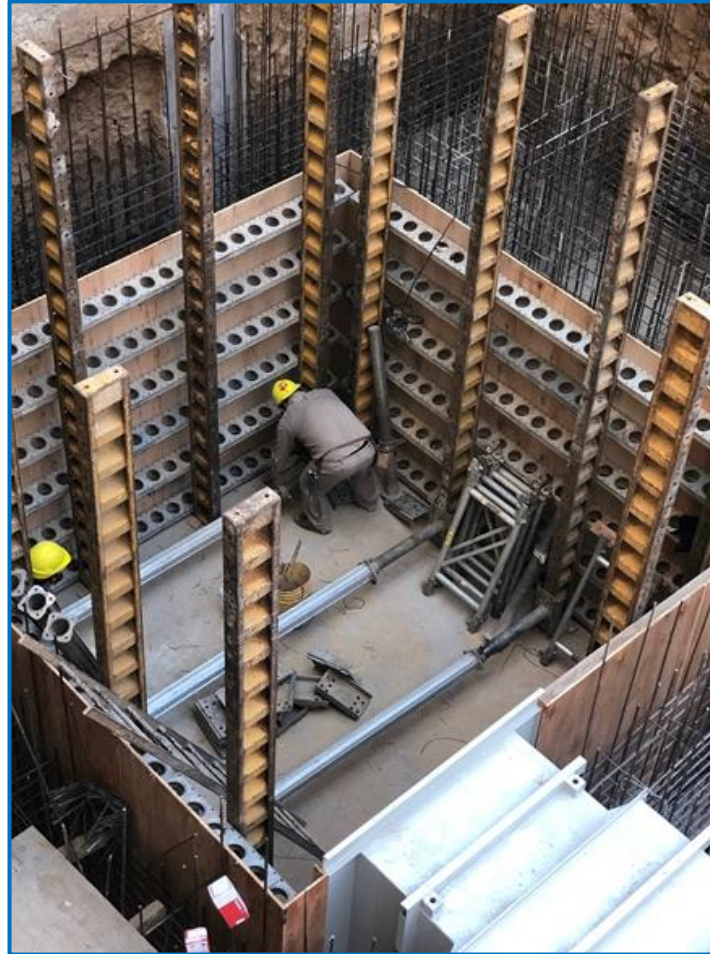
Shoring system to intern vault wall
