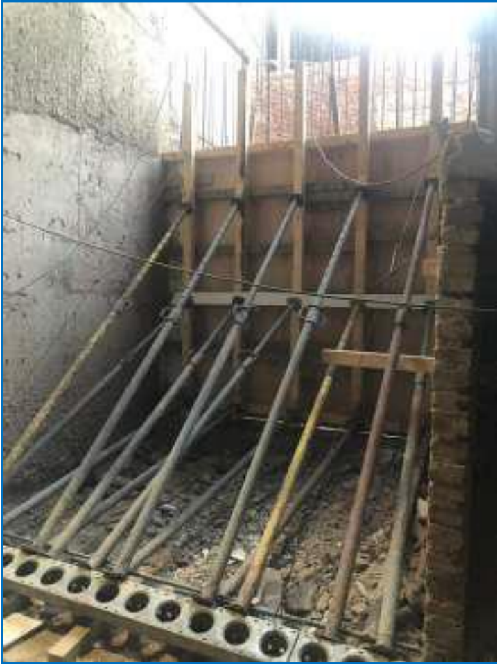
Shoring system to extern vault wall
