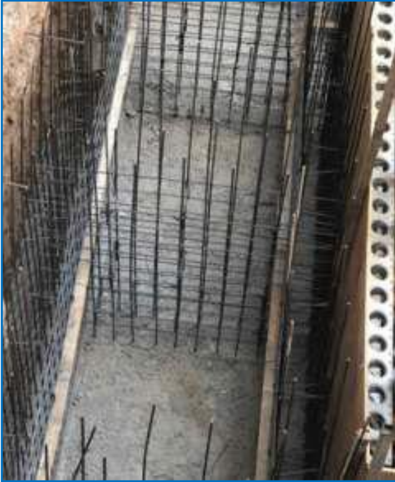
Wooden frame inside the armor previous the concrete cast
