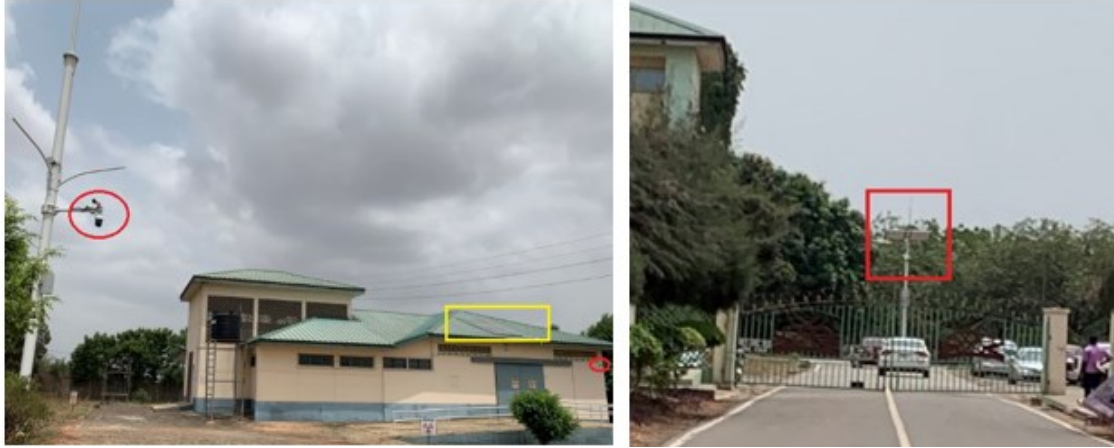
Fig. 4. Outside security features of the CDSRSSF and GAEC site
