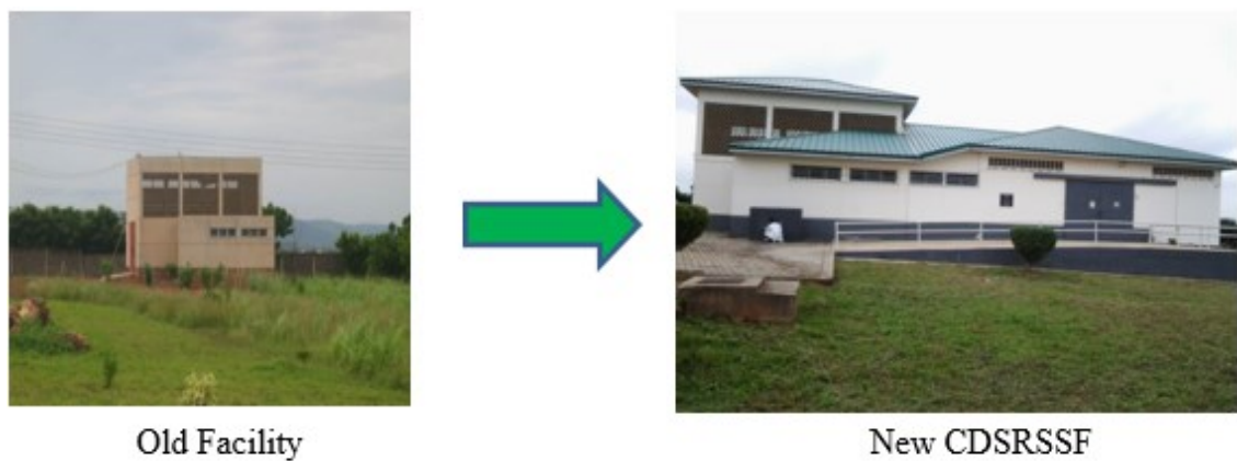
Fig. 2. Transformation of radioactive storage facility
