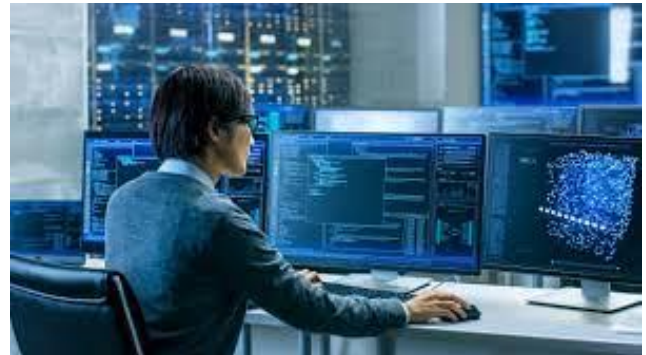
New central alarm station
