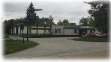
Photo of the Irradiation Facility
