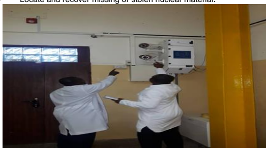
Assessing camera effectiveness at a facility
