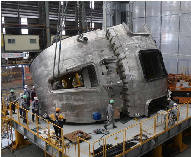
<Segment Setting for Final Assembly>
