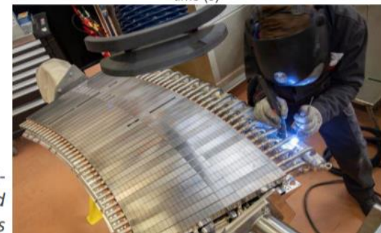
Welding of a 30 degree-sector of divertor composed of 38 ITER-grade PFUs
