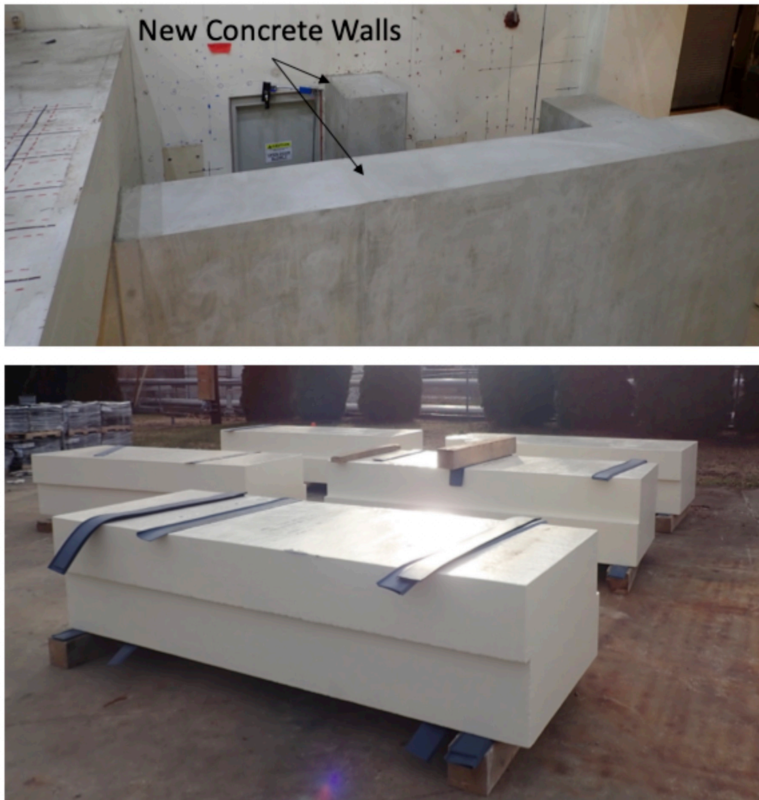
Figure 3: Figure 3: New shield wall (top) and roof blocks (bottom)
