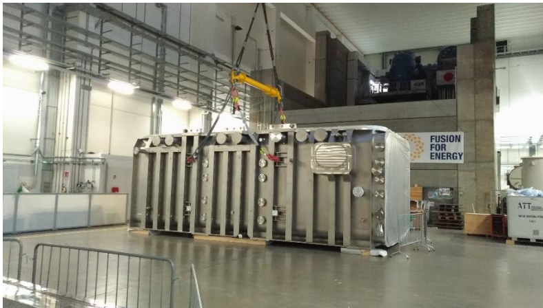
Delivery on site and installation of the MITICA BLV
