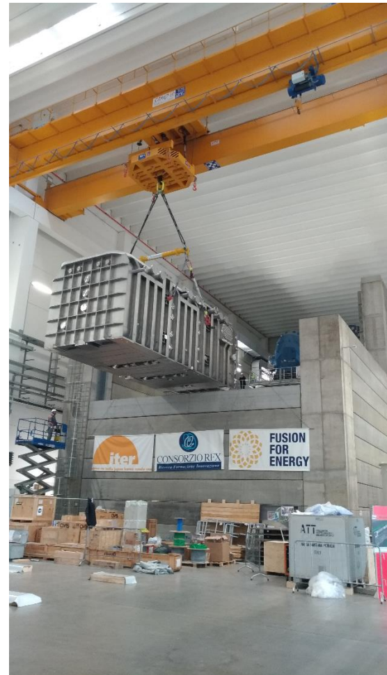
Delivery on site and installation of the MITICA BLV
