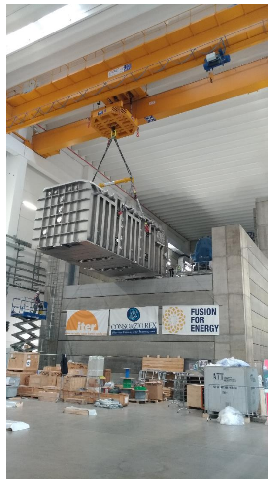
Delivery on site and installation of the MITICA BLV
