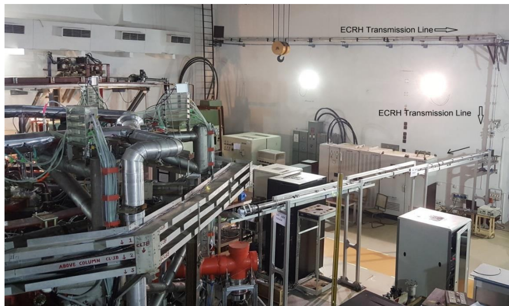
ECRH System in ADITYA-U tokamak
