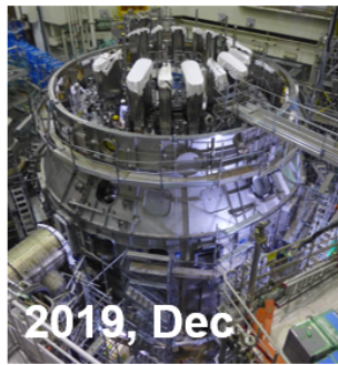
Cryostat Vessel Body
