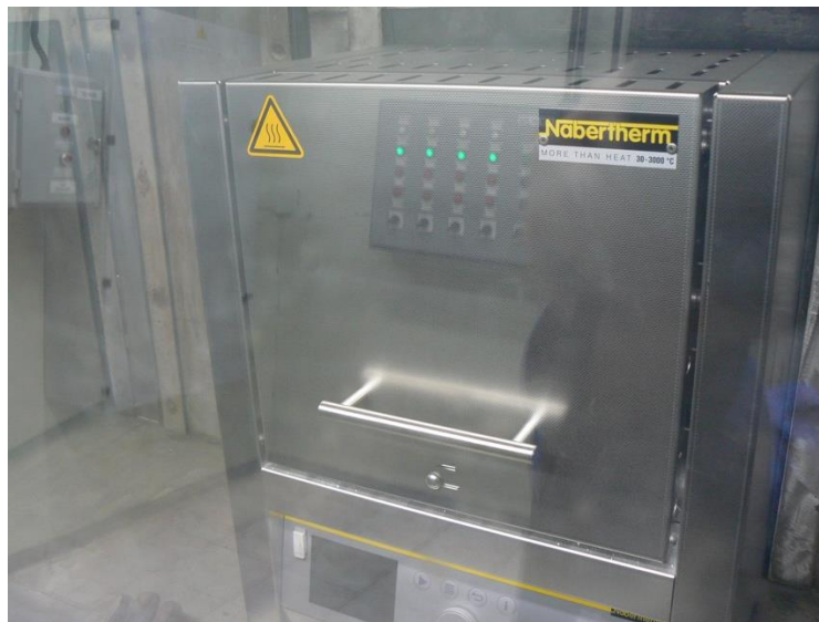
Fig. 4. Newly installed Nabertherm Furnace
