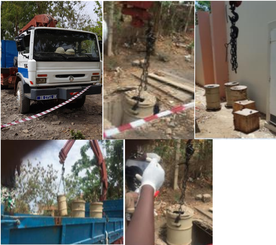
FIG.5. Vulnerable radioactive sources removal from facility
