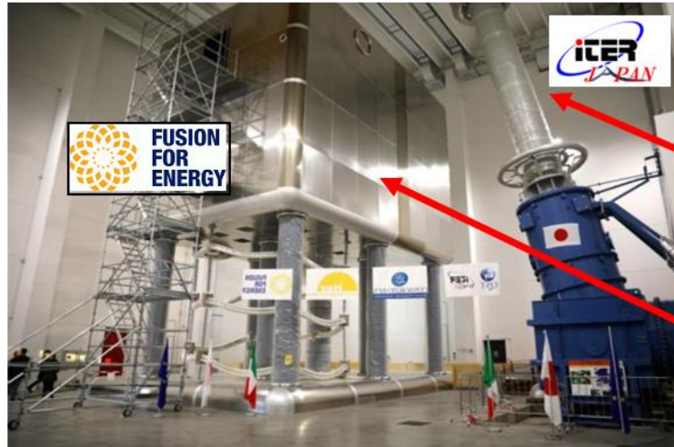
Fig. 10. 1MV Faraday Cage (hosting Ion Source PS)
