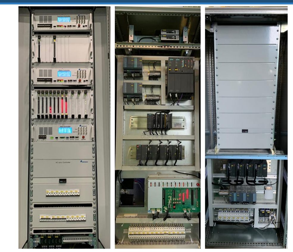
Fig7. Conventional/Interlock/Safety cubicle
