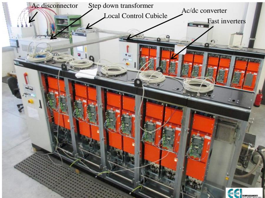
FIG. 4. Arrangement of the whole RWM-PS system for the final integrated tests
