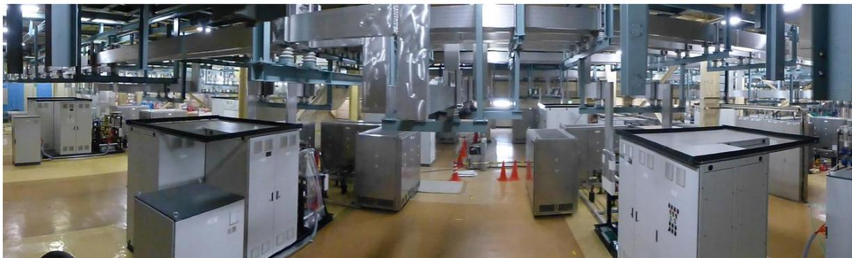
FIG. 2. Panoramic view of some Quench Protection Circuits after installation in one Power Supply hall at Naka site.
