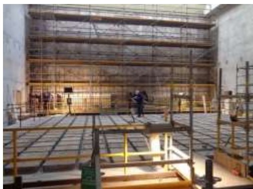
Fig. 3. Atucha Dry Storage Building
