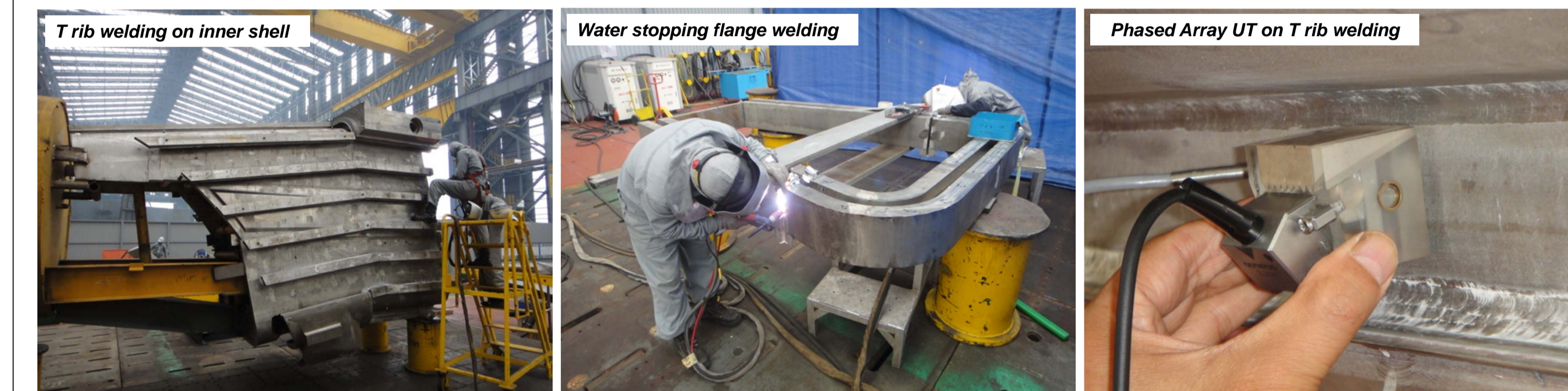
Fig. 5. Fabrication status of lower PSE full-scale mock-up
