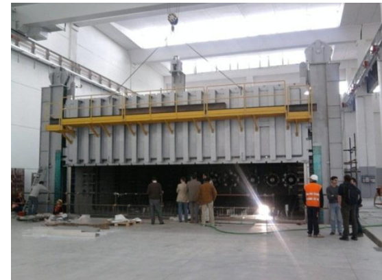
Heat treatments furnace
